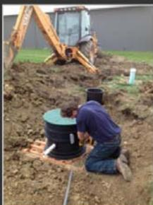
Ray Tebo, of New Excavating Technologies, installs Will County's first BioBarrier membrane bioreactor wastewater system in the Old Plank Industrial park in New Lenox. | Susan DeMar Lafferty/Sun-Times Media
