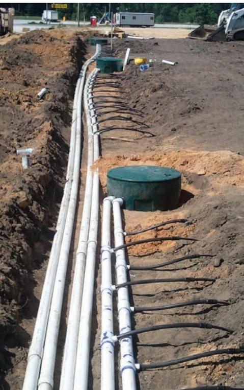
dictated that we set the septic tank at an elevation that precluded flow by gravity, which is why we needed a lift station pumping to the flow equalization tank,” says Rexroth.
