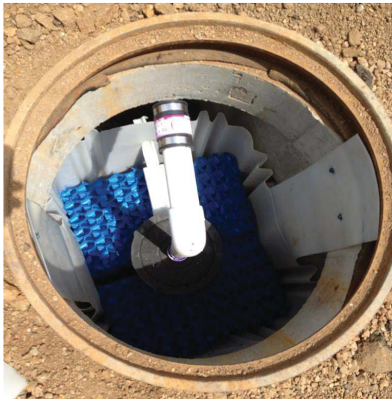
A RetroFAST system is inserted into an existing manhole.
