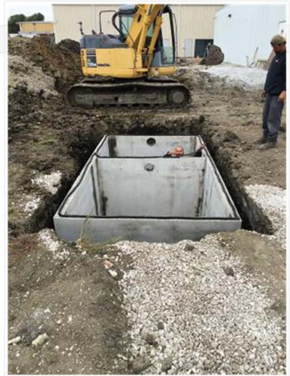
Technician Jim Koltunchik applies ConSeal butyl sealant on the Wieser tank for the MBR at the Dwight, Illinois, marijuana processing operation.
